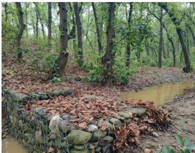
LOOSE BOULDER STRUCTURE CONSTRUCTED AT BELWALI VILLAGE
